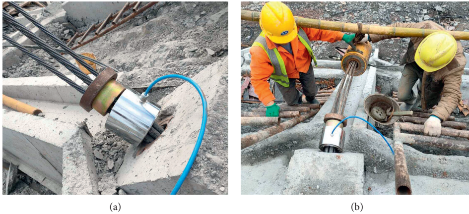
FIGURE 3: Installation of the anchor cable meter.
