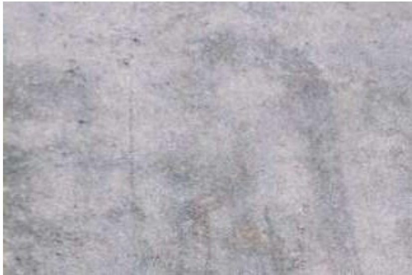
Fig. 5. Effect of rainfall on the in situ concrete
