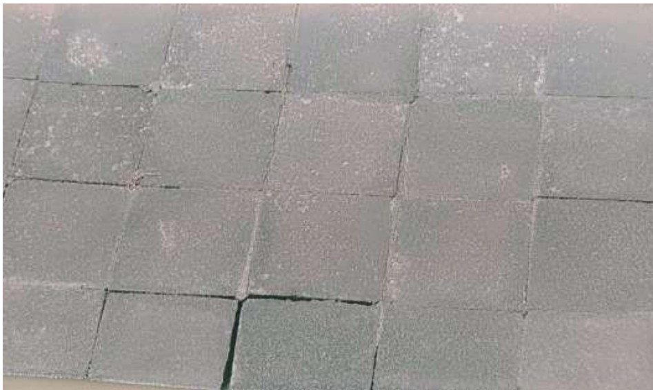
Fig. 8. Removal of joints between the joints of precast concrete
