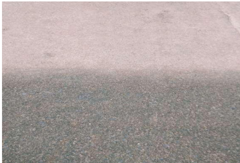
Fig. 3. Observation of concrete face above and below the free board
