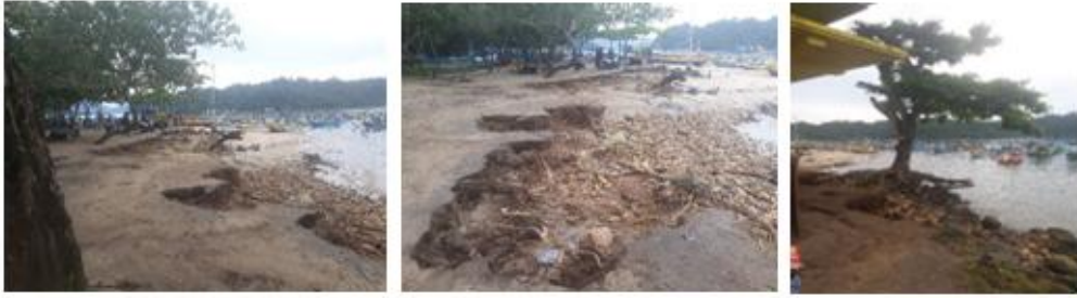
Fig. 12. Photos of the abraded condition of Sendang Biru Beach
