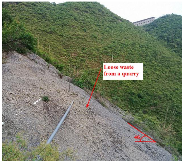
Fig. 7. Loose slag from the quarry
