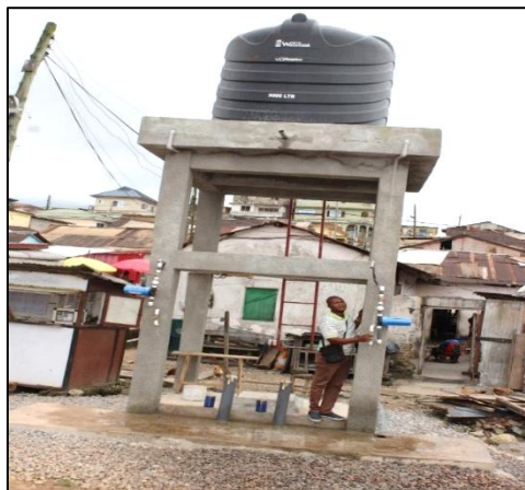
Fig. 4. Private Borehole at Mgbushimini Neighbourhood as Source of Water Supply
